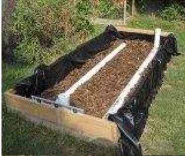
The beds must be level so that the depth of the water is the same throughout the bed.
